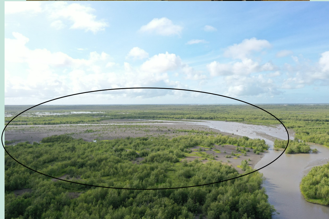
Sediment trapping unit and planting of young Mangrove for Mangrove rehabilitation and conservation
